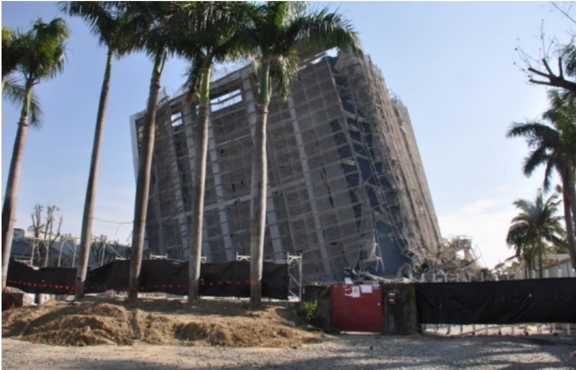
Figure 9. A new building nearing completion tilted severely after the 2016 Meinong earthquake (Hsu, 2022a).
